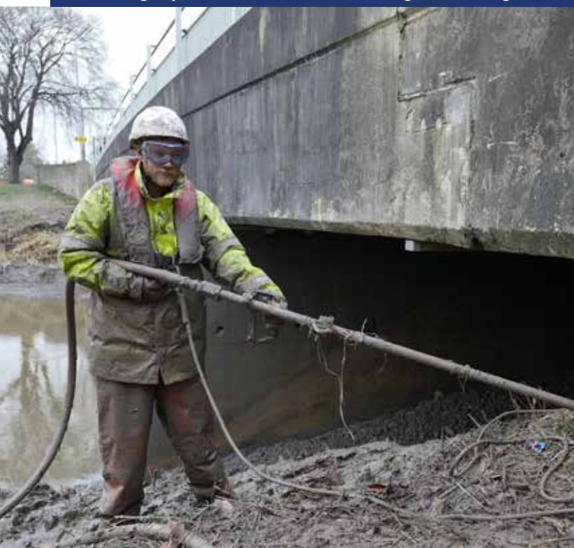
De-silting operations at Blake Bridge in Bridgwater
